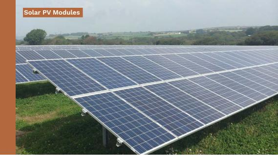
The areas marked as 'developable' will include solar photovoltaic (PV) modules that will convert sunlight into electrical current. We are proposing that each solar module will be approximately up to 2.5m long and 1.3m wide. The modules will each consist of a series of PV cells beneath a layer of glass. Each module will make up a single solar panel.
