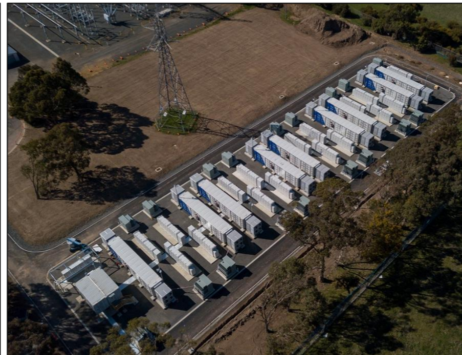
Typical battery storage compound configuration
