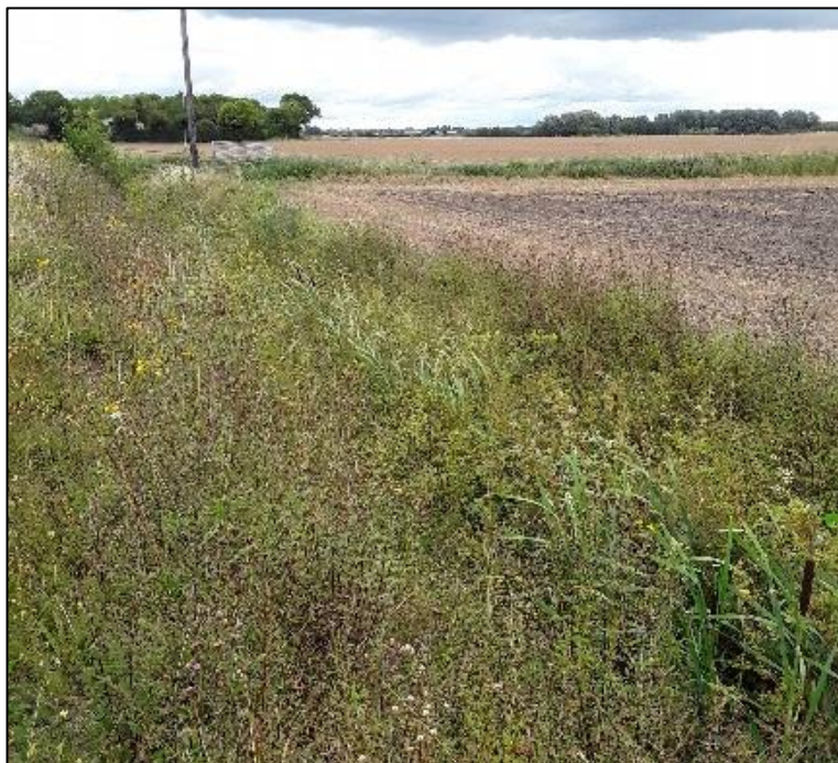
Plate 8D-17: Ditch 09 on Ness Road
