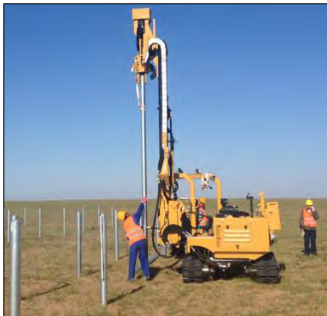
Plate 3-15. Piling of module mounting structures.
