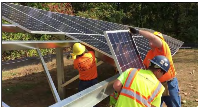
Plate 3-16. Construction staff mounting solar PV modules by hand.
