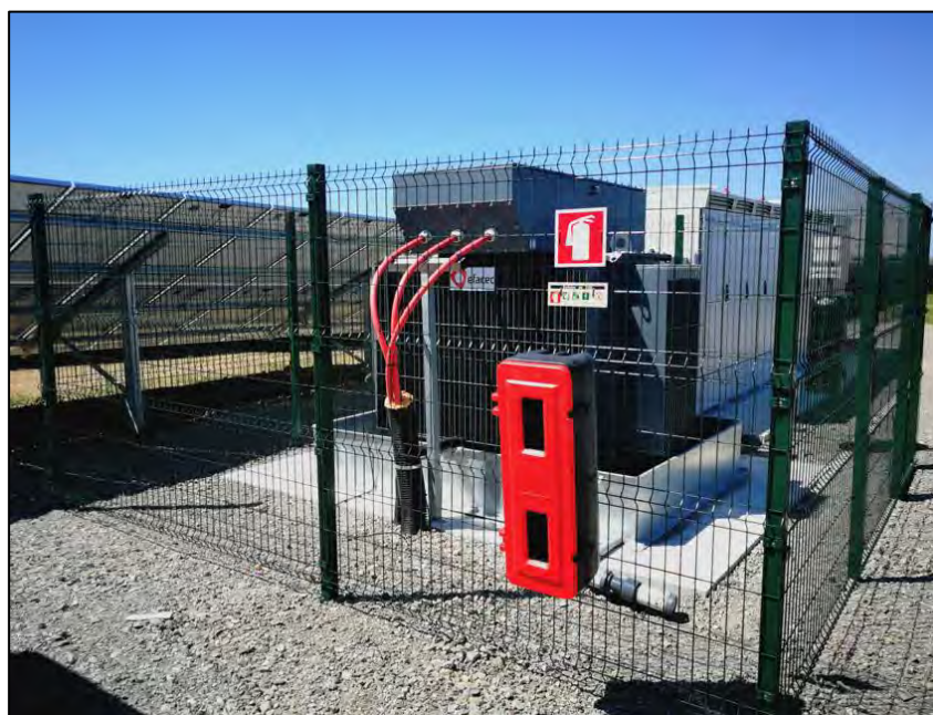
Plate 3-12. Typical transformer compound fencing
